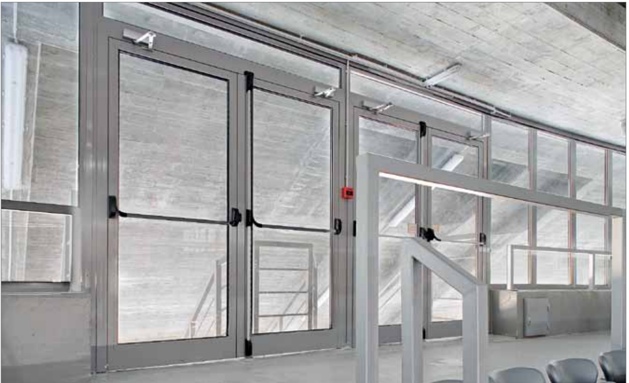
Sports Hall, Zadar, Croatia (Photo: Robert Les)
