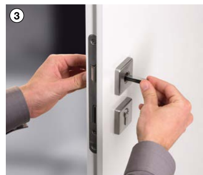
3 Insert the solid profile spindle
