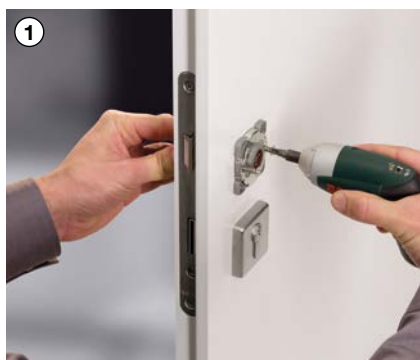
1 Place the base and tighten the screws
