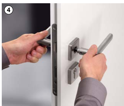
4 Put the door handles together and tighten the grub screw
